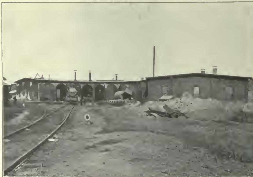
FIG. 662. FACILITIES TO BE ABANDONED. Locomotive engine house of the Chicago & North Western Railway, near 14th Place and S. Robey Street. This building has 12 stalls, each 64 feet long, and is of an early type of construction. In the event of electrification, it would be rendered worthless to the railroad.
